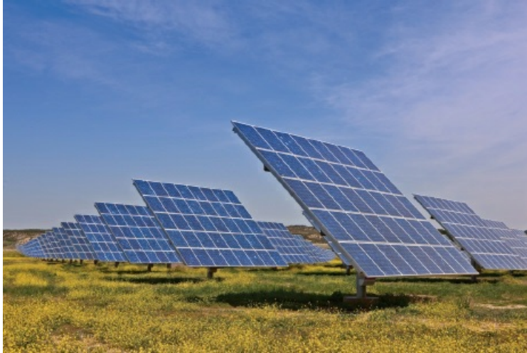
Figure 1.26 Ground-mounted systems in a solar farm
