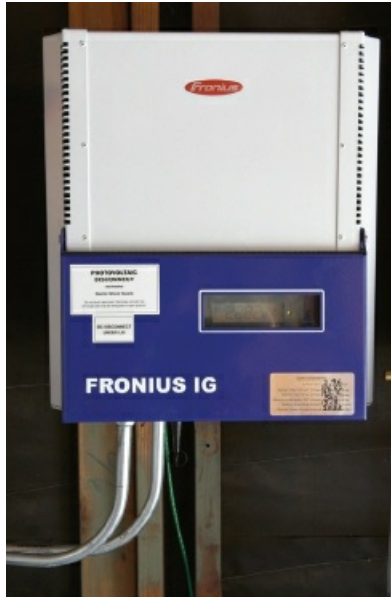
Figure 1.27 Photovoltaic inverter
