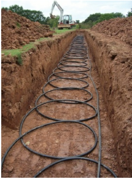
Figure 1.15 Slinkies being installed in the ground
