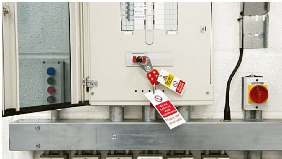
Figure 7.13 Isolation of an installation should be part of a planned and agreed procedure
