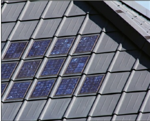
Figure 1.24 In-roof mounted system
