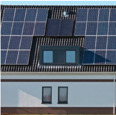
Figure 1.29 Building features shading a photovoltaic system
