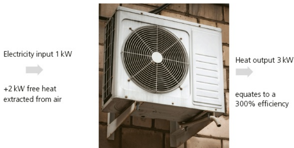
Figure 1.10c The efficiency of an air-source heat pump
