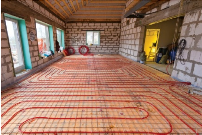
Figure 2.118 Electric underfloor heating before the final screed is laid
