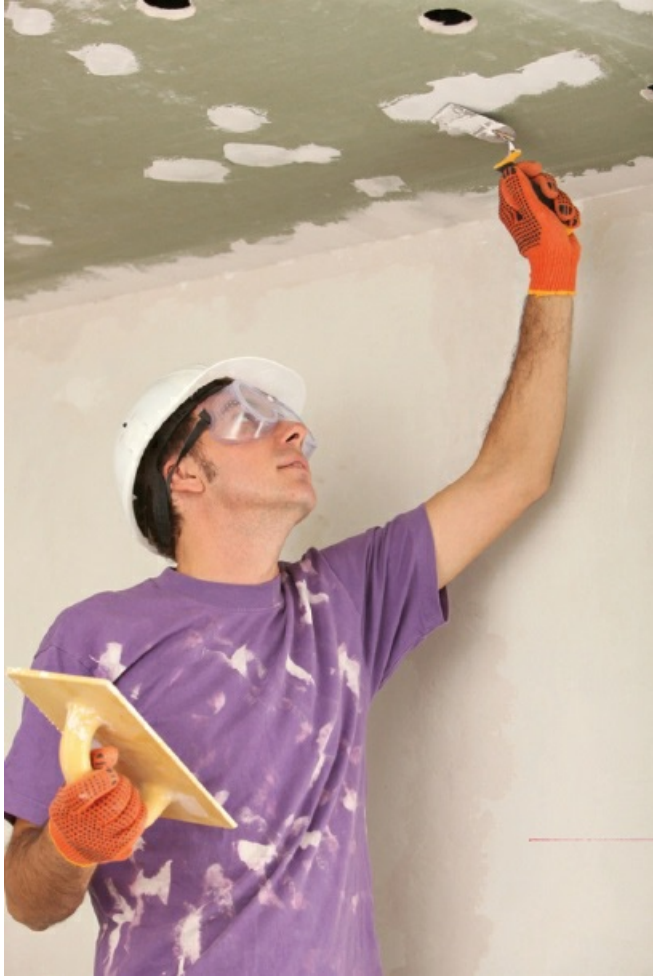
Figure 4.14 Repairing a hole in plasterboard
