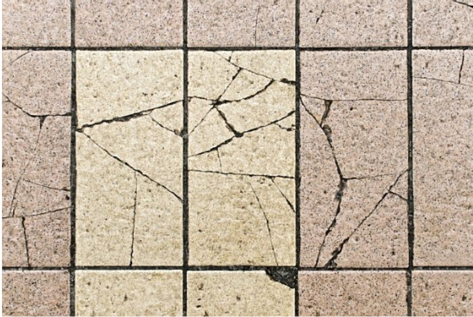
Figure 4.17 Damaged wall tiles
