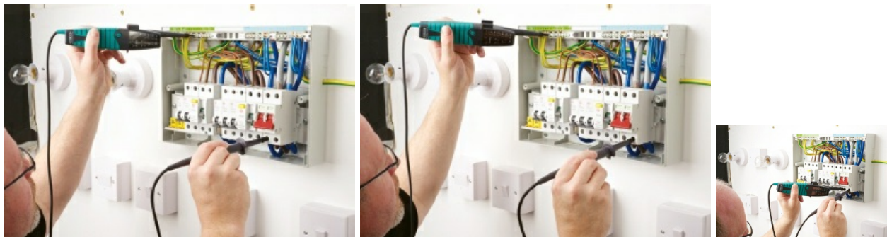
Figure 7.15 Checking the supply voltage
