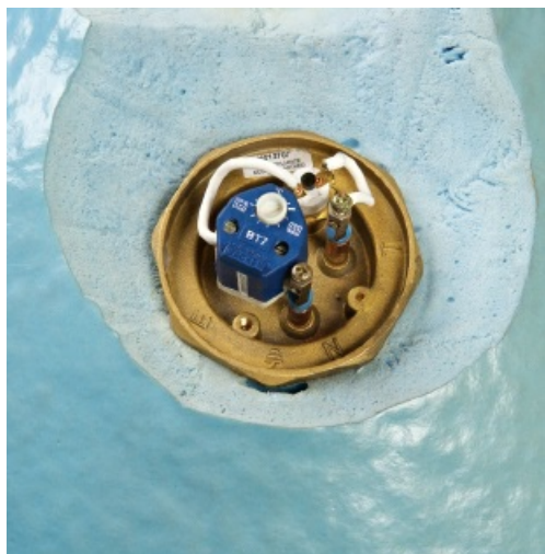
Figure 2.124 Thermostat inside pocket in heater element
