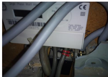
Poorly positioned customers RCD with broken cover. Terminals now exposed to touch.
