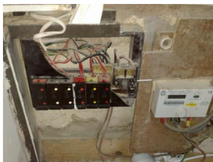
Customer's old Wylex consumer unit with severely damaged cover, exposing live terminals
