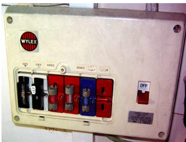
Exposed live fuse carriers and consumer unit lid missing – also 13a BS 1363 fuse in lighting circuit
