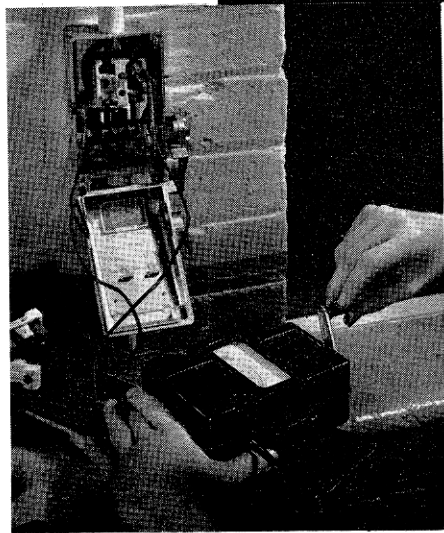
Figure 11 Making an insulation test at a switch-fuse
