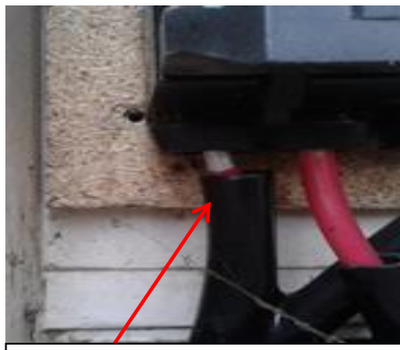
Example of exposed live conductor where the insulated trousers have slipped exposing the live conductor
