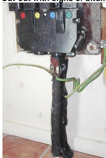
Cut-out with signs of bitumen leaking
