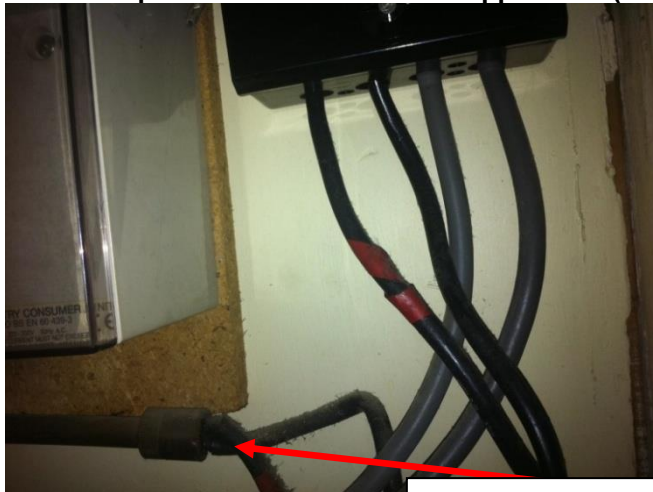
Example of Mineral Insulated Copper Clad (MICC) cable
