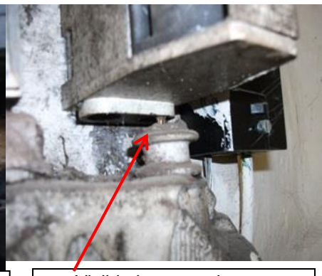
Visible bare conductors
