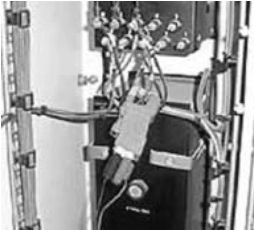
Figure 4. Small Clip-on CT Around the Secondary of Existing Instrumentation CT.
