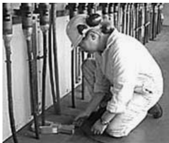
Figure 3. Clip-on CT Around Supply Cable.
