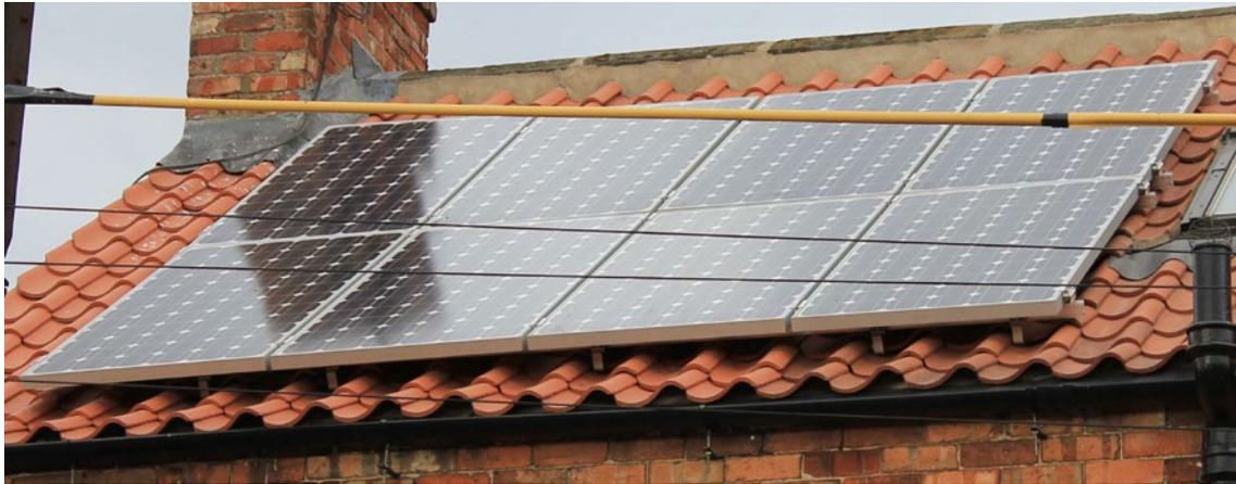
When solar panels are installed within a property it is always necessary to have them aligned with the sun in such a way that the maximum amount of solar radiation will fall on the panels. For example, there is very little point in Britain of installing a solar panel array on a north-facing wall or roof. The amount of sunlight is severely restricted and the cost of installing the panels would never be recovered.
