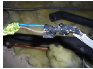
Connections likely to cause a fire
