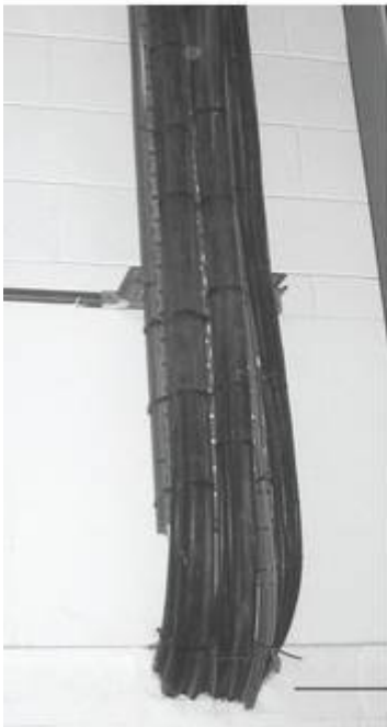
Heavy duty traywork used to support groups of SWA cables
