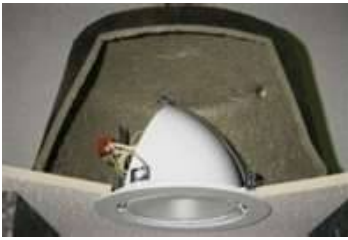
Firehood fitted to a downlighter
