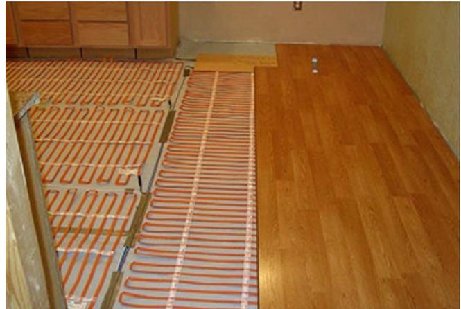
The heating cables themselves are made from a range of substances. Chromium, aluminium, copper, silicon and manganese alloys have all been used. The insulators used include asbestos, mineral insulation, butyl, silicon rubber and nylon. All of these insulators are usually covered with a plastic sheet to protect them from damage.
